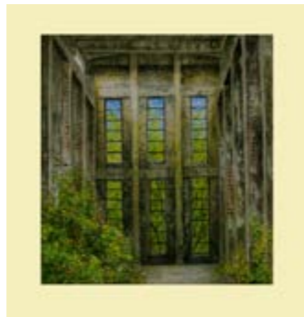
THE LIQUID OXYGEN FACTORY; Echoing with birdsong, low sunlight dappling raw concrete and shattered plaster walls in bright, flickering shadows, it is reminiscent of some vast Brutalist cathedral.
