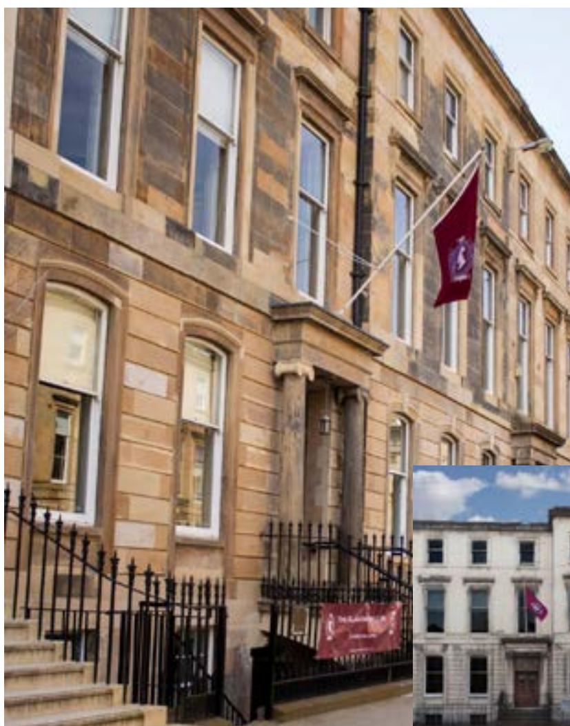
Dramatic improvement in the building's exterior
